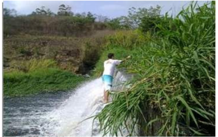
Andre hard at work clearing the reeds at the wall
